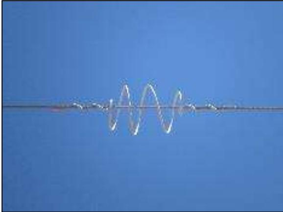
**Photo 1** Bird diverter on the earth-wire
